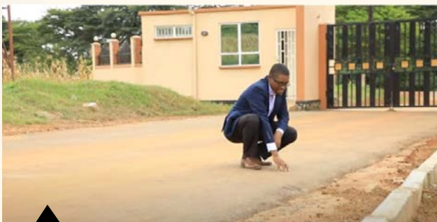
Above: The Director of Graduate Studies, Prof Samson Rwahwire, inspects the road works
