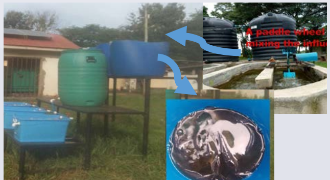
Figure 3: Effluent rich in microalgal bacteria floc biomass and dissolved oxygen concentration from the paddle wheel mixed HRAP used as a feed for the fish tanks in the aquaponics system to improve catfish growth. Catfish weight increment from 2g at stocking to 36g after 12 week monitoring period was recorded.
