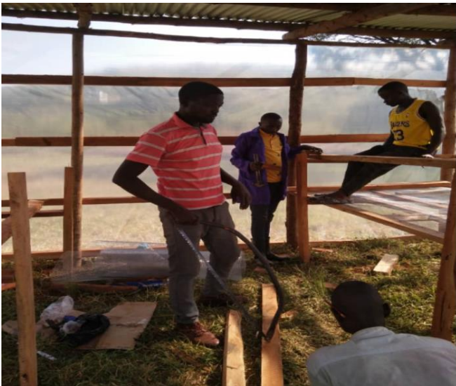
Students constructing a drying shade
